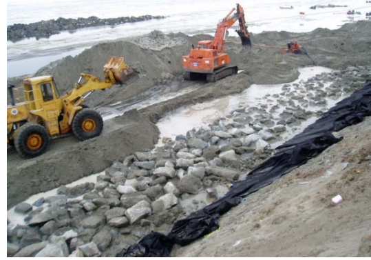
Kawerak Transportation project in progress.
